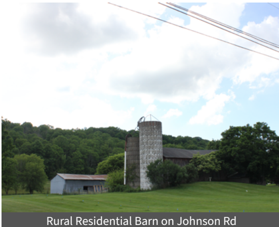
Rural Residential Barn on Johnson Rd
